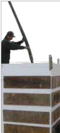
Some competitive ICFs strap corners with lumber for strength during concrete placement.
