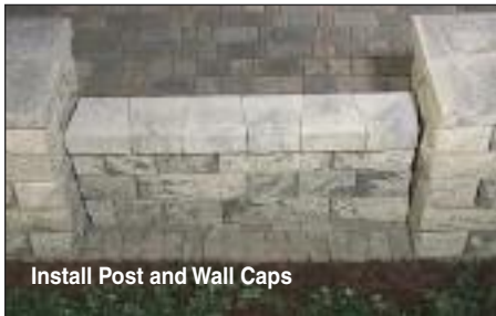
Finish wall panel to desired height.
