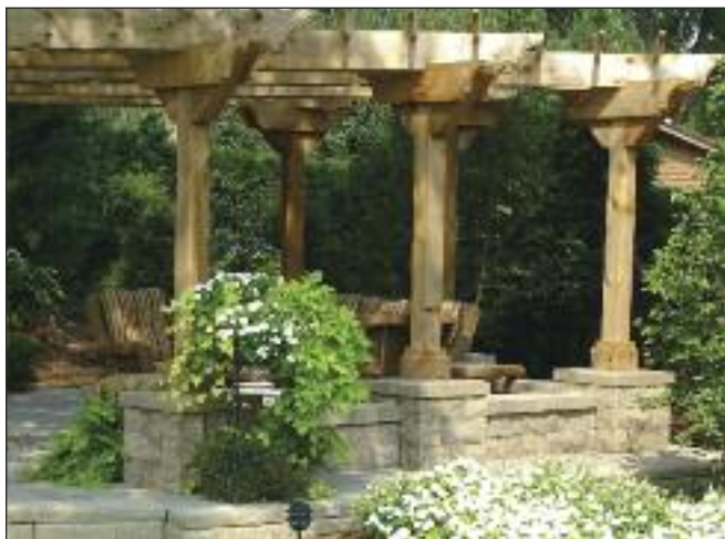
Built on existing patio
