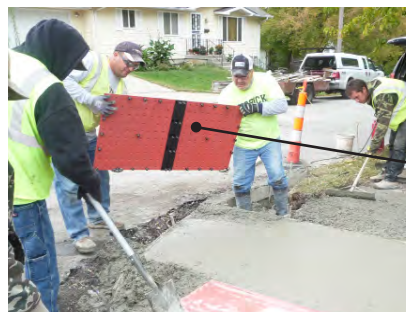
Simplify Wet-Set installation by connecting panels.
